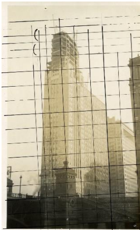
Fig. 3 Bernard Boutet de Monvel, Chicago Landscape - London Garantee Building , vintage photograph squared for transfer, 1928. Stéphane-Jacques Addade collection
